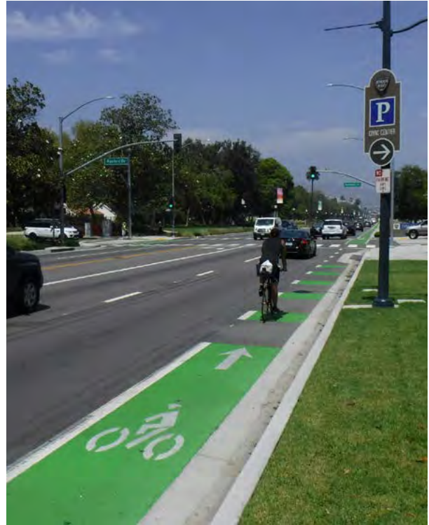
An example of green painted bike lane with skip boxes at merge areas where there could be a conflict between vehicles and bicycles.
