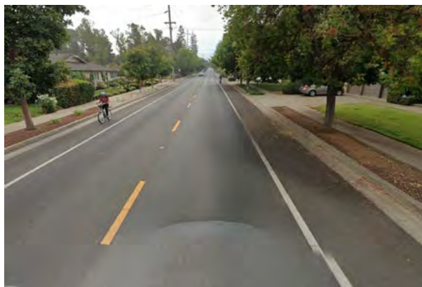
Los Altos Avenue looking south. Bicyclists use the on-street parking lane when available to avoid vehicles moving at higher speeds.
