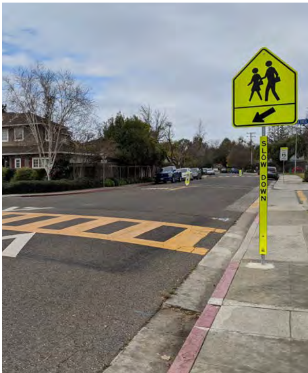
High visibility crosswalks painted in yellow with school crossing signage and a raised crosswalk have been installed in front of Springer Elementary.
