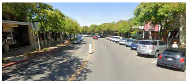
Main Street looking north. Main Street has parallel and angled parking, one vehicle travel lane in each direction, curb extensions at intersections, and decorative crosswalk markings.
