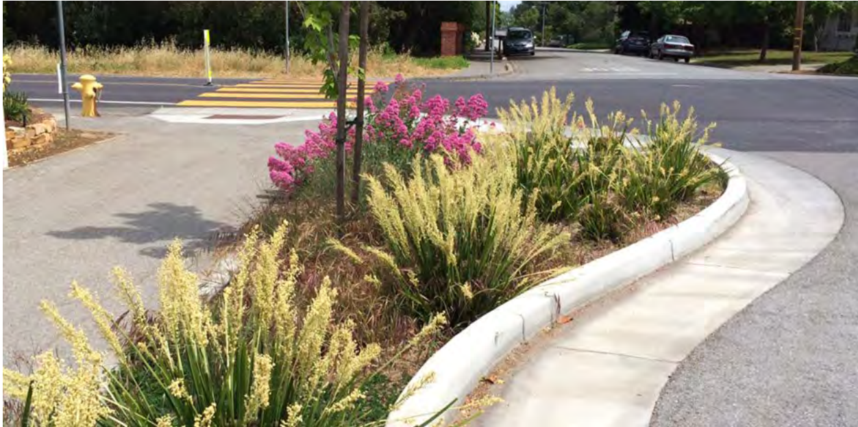
Green Stormwater Infrastructure can take many forms such capturing water runoff from the road in curb extension planting beds shown in the image above.
