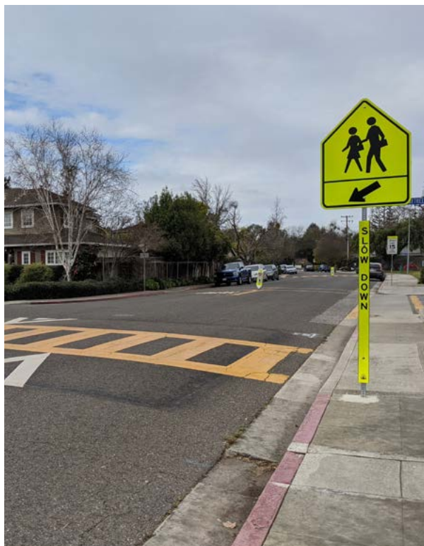
High visibility crosswalks painted in yellow with school crossing signage and a raised crosswalk have been installed in front of Springer Elementary.
